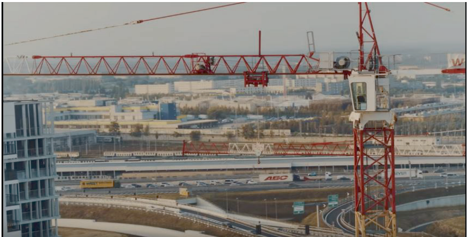
Fig. 1. Construction site with a crane in Capo Plaza, Giovane Fuoriclasse (1:57)
